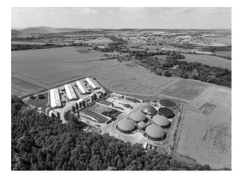
The waste is stored and allowed to decompose producing heat and useful gas. If it gets too hot it presents a fire hazard, so a warning system is required.
